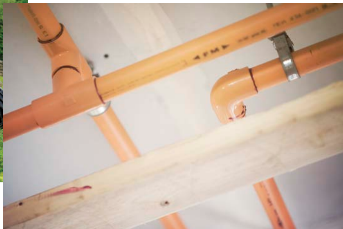
In an ISO-compliant, peer-reviewed lifecycle assessment, our BlazeMaster® fire sprinkler systems were found to have half the climate change impact of steel.
